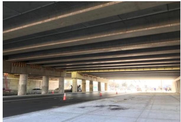
Peoria Street after 12-foot wide shared-use sidewalks are installed on the east side. The west side has 8-foot-wide walkways.
