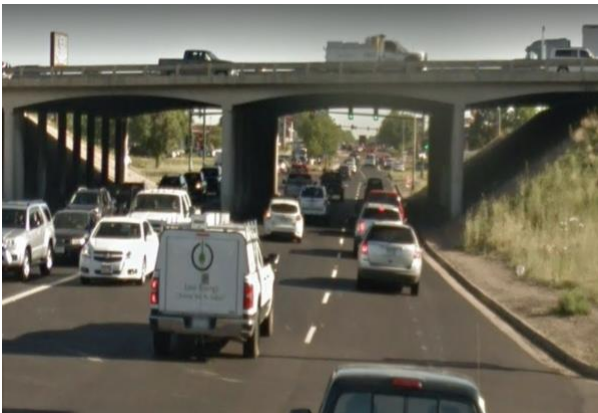
Peoria Street before construction in 2017.
